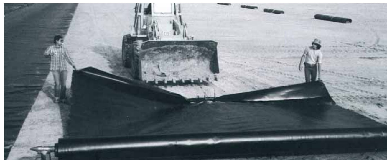
Posa in opera
