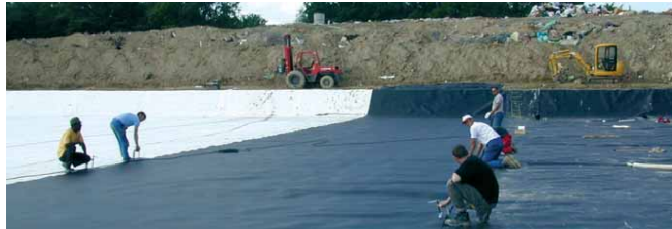
Posa in opera
